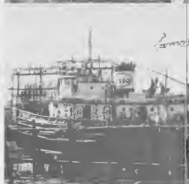
THE ESSO Oranjestad is positioned on keel and block as she goes into drydock. A diver, above, prepares to descend to check the condition of the drydock tracks as a workman washes off the chains to keep the hauling engine from becoming fouled.
